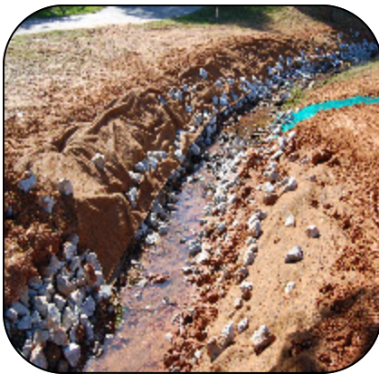
Erosion control work gets underway
